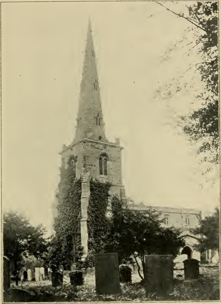
CHURCH AT PODDINGTON, BEDFORDSHIRE, ENGLAND
